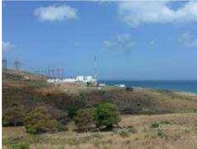
Figure 17 : Station ONEE " Branche Electricité
