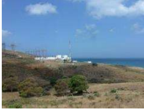
Figure 20: Station ONEE " Branche Electricité"
